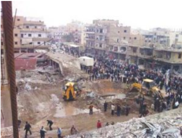
Destruction in 23 February Street after the rocket attacks of November 2013
